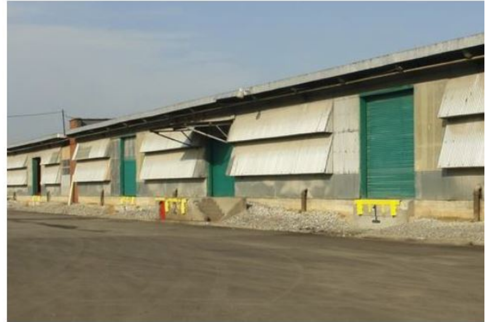
Functional Industry (No Office Rehab Potential)
