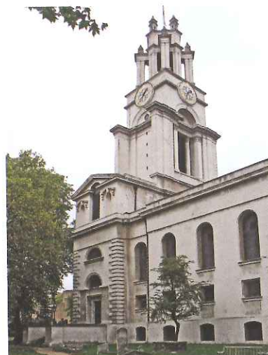
Above: St Anne, Limehouse
