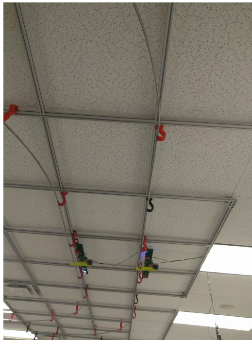
Figure 1: A picture of the overhead track and the gate
